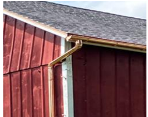
Barn Gutters (Installed August 2025)
